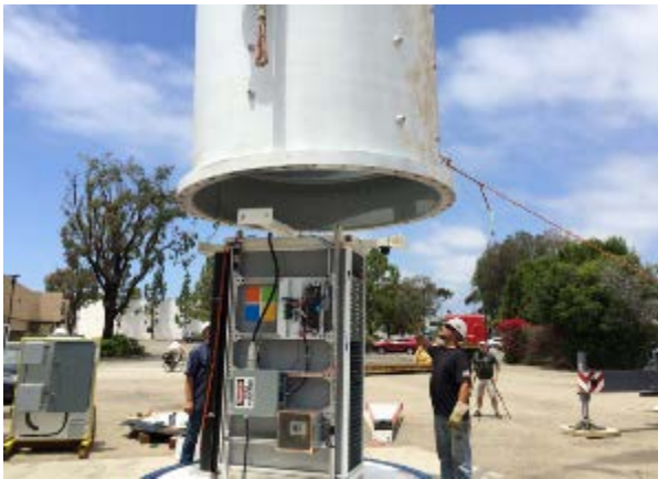
Figure 47. Microsoft Project Natick – modular submersed server with ocean cooling, San Luis Obispo, California. Source: Microsoft
