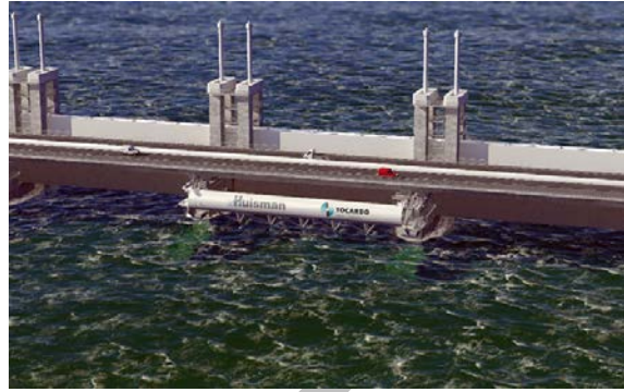
Figure 58. Five tidal turbines integrated with the Oosterscheldekering storm surge barrier in the Netherlands. Photo from HydroWorld.com
